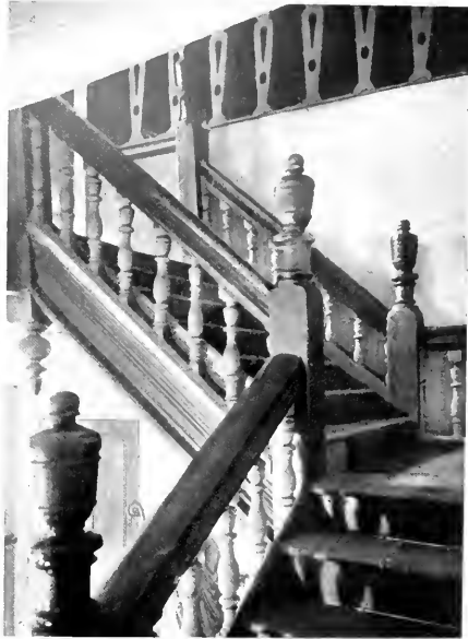
151. Staircase, Boleyn Castle.
